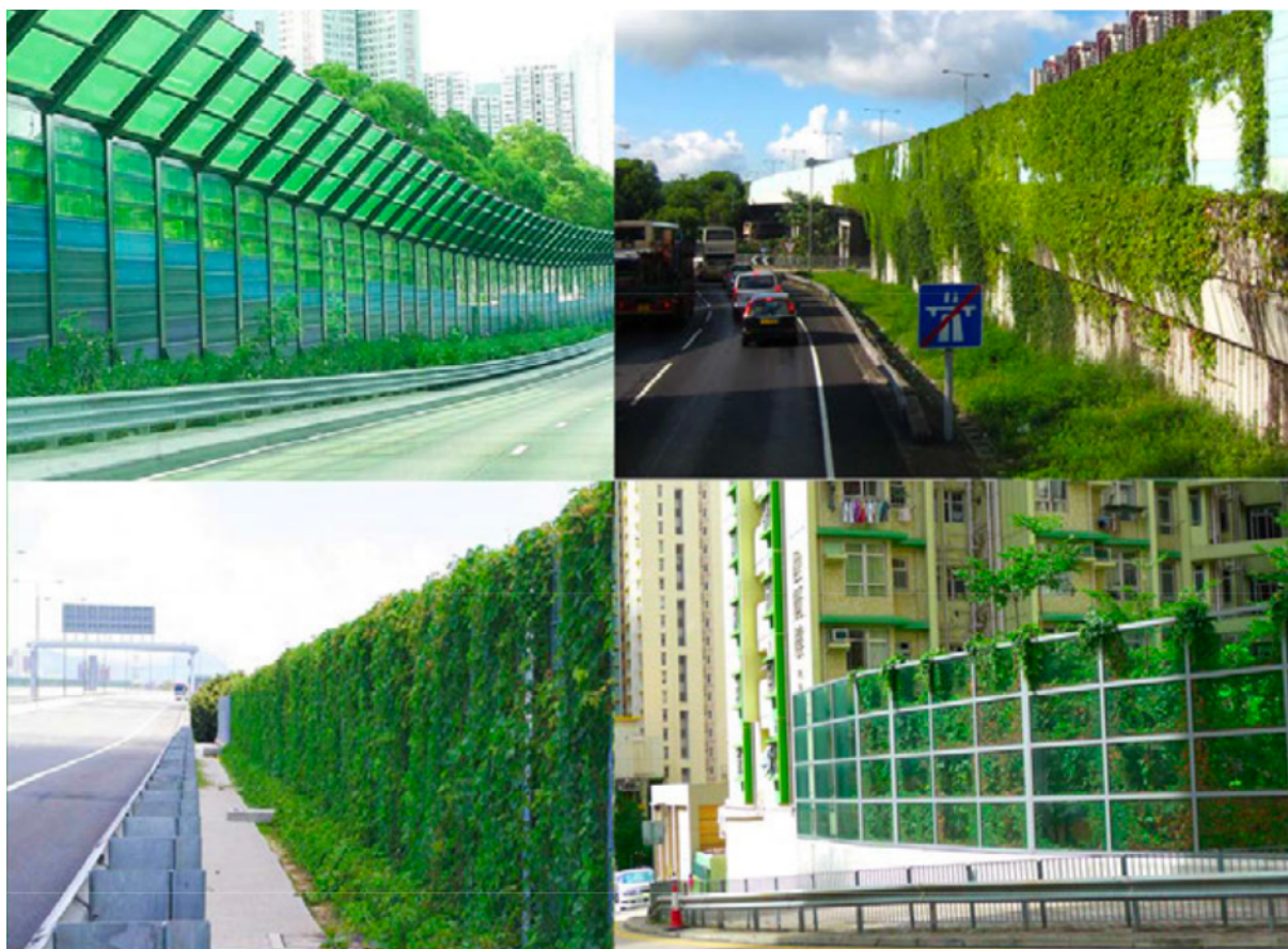
Figure 7: Visual screening provided by “green” noise barriers in Hong Kong
